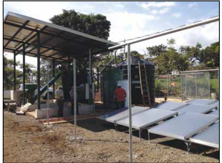
Actual solar-powered anaerobic digestion system being installed based upon student design work, Fabio Baudrit Experiment Station, Alajuela, Costa Rica.
