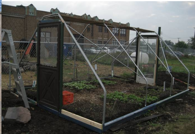
12' wide, 12' long, ~ 7' tall; 10' long 1" diameter EMT conduit bent at 45° and joined at top. Exterior joining spline and ground posts made with 1.3" chain link fence top rail.
