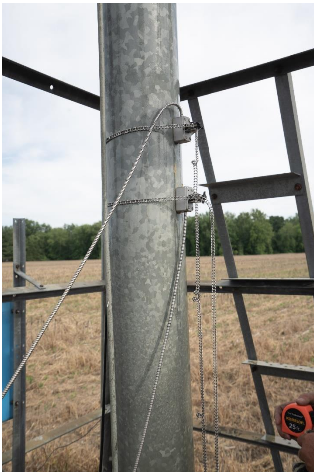
Pressure gauge & Doppler flow meter (Flow and Pressure Measurement)
