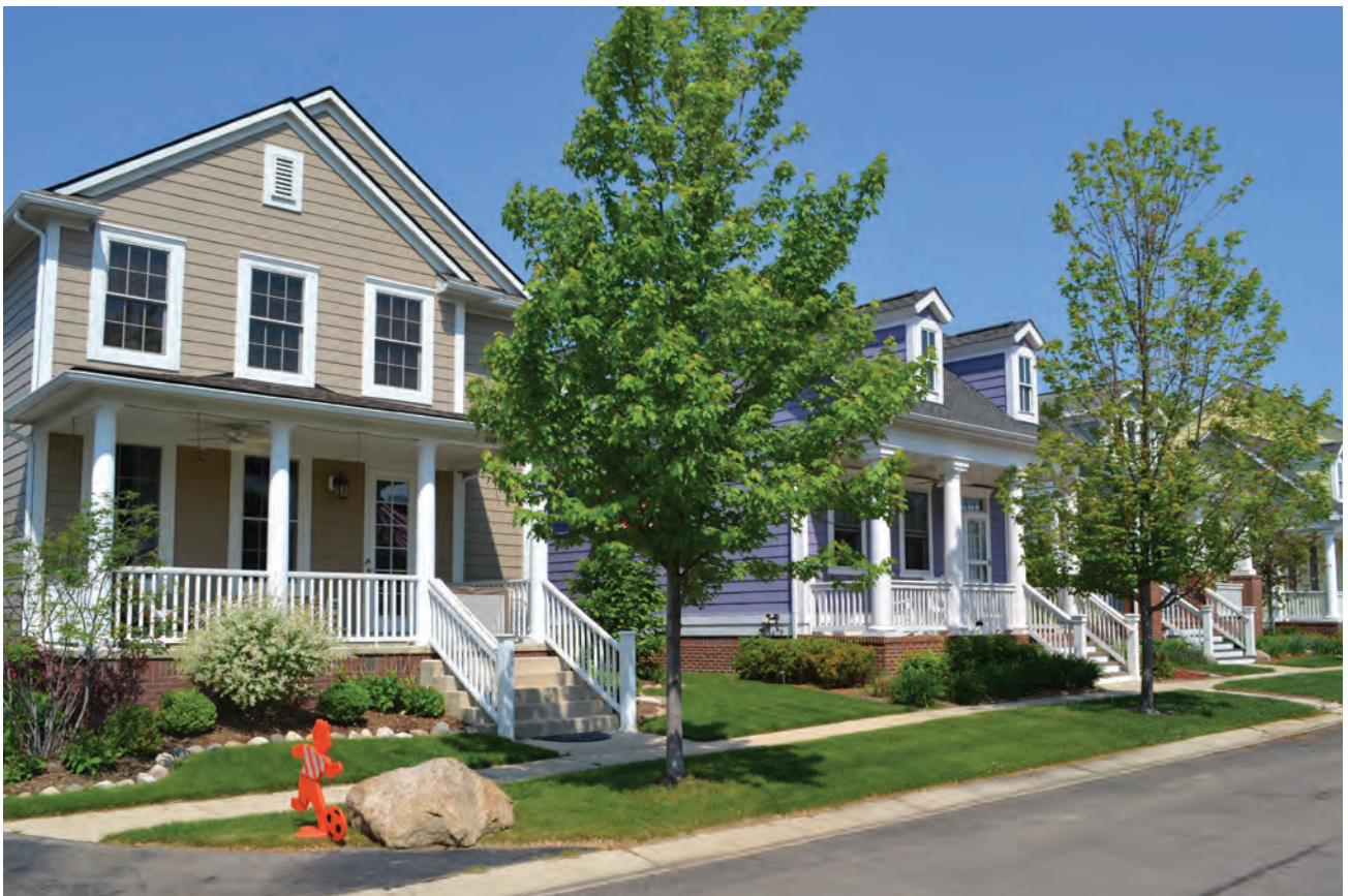
Cherry Hill Village in Canton, MI. A neighborhood built on New Urbanist principles. Photo by the MSU Land Policy Institute.
