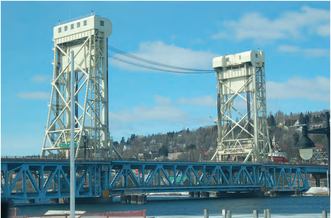
The Portage Lake Lift Bridge connecting Houghton and Hancock, MI. Adjacent cities present unique opportunities for joint placemaking. Photo by Kurt H. Schindler, AICP, MSU Extension.
