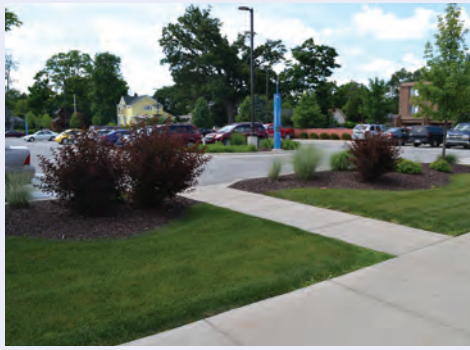
Landscaping breaks up large areas of pavement and allows for some stormwater infiltration.
