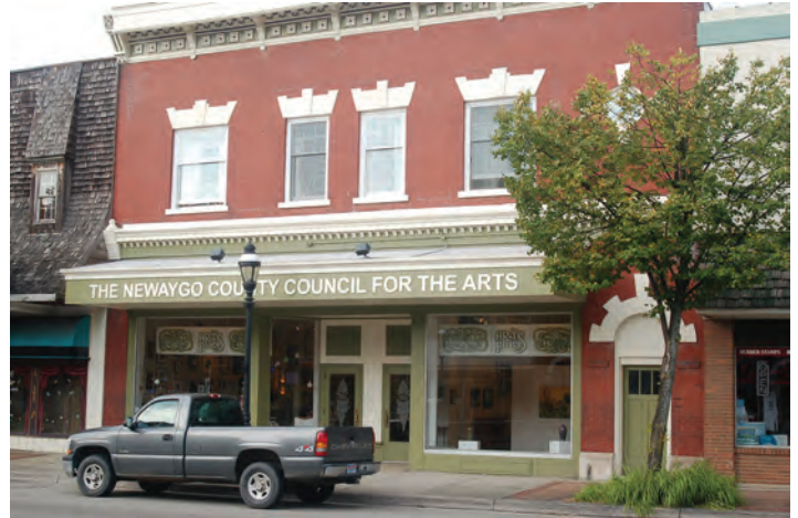
Historic building in Fremont, MI, which utilizes a form-based code. Photo by Kurt H. Schindler, AICP, MSU Extension.
