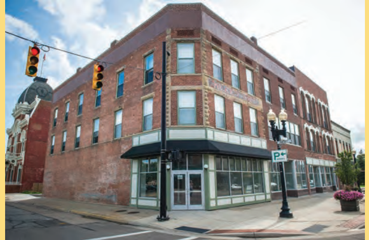
The Kerr Building, nearly completed after redevelopment. Photo by Derek Booher, for the City of Coldwater.
