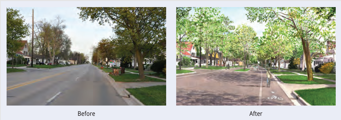
Figure 6–9: Before and After of Local Street on a Road Diet – City of Williamston
