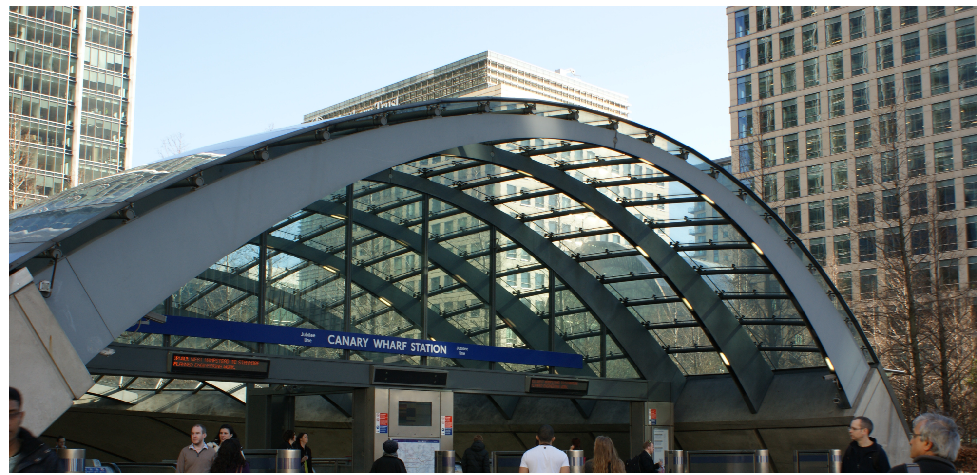
THIS DETAIL RESEMBLES THE OVERALL APPEARANCE OF WHAT THE ROOF OF THE AMPHETHEATER WILL LOOK LIKE
