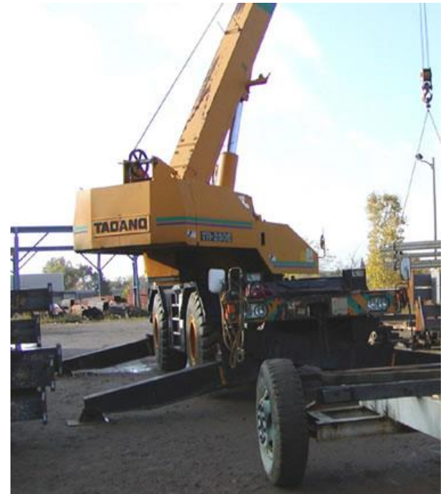
Mobile crane used to load material for shipping
