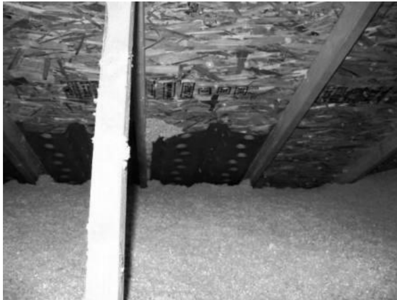
Figure 5.5: Attic Ventilation Baffles (source: http://www.peaktoprairie.com/?D=206 )
