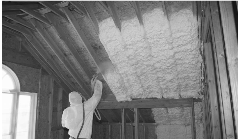
Figure 5.4: Spray Foam Insulation (source: http://www.certainteed.com/products/insulation/spray-foam-insulation )
