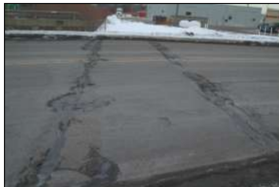
Figure 35 – GrandWalk Trail Intersection at Alpine Avenue
