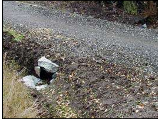
Figure 42 – Crushed Rock Surface
