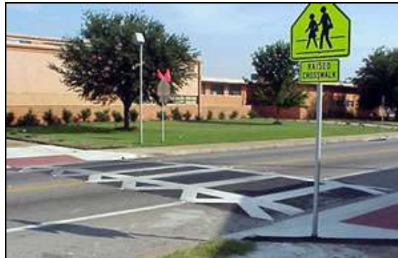
Figure 34 – Example of a raised crosswalk
