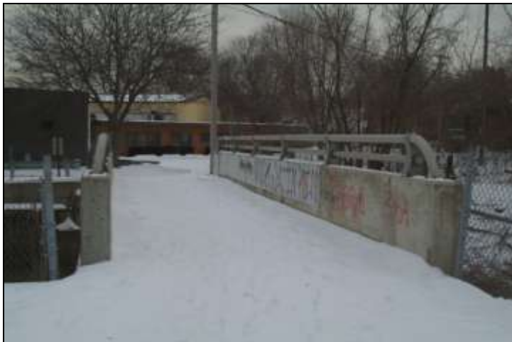
Existing Pedestrian Bridge Over Indian Mill Creek
