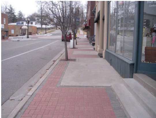
Picture 10: Newly Improved Sidewalks along Bridge Street
