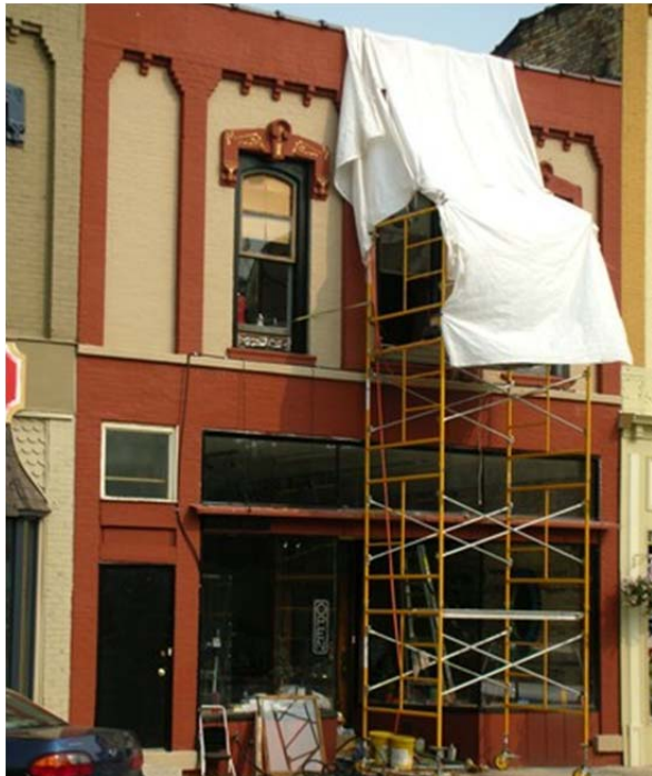
Figure 12 - Renovating Building Facades
