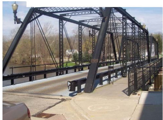
Figure 10 – Iron Truss bridge in downtown Portland
