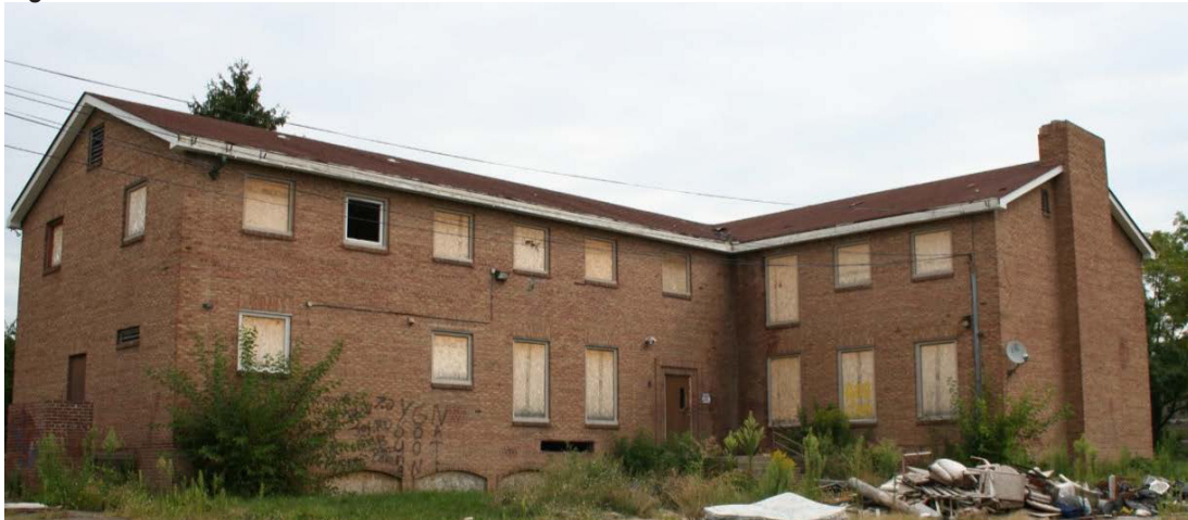
St. Peter's Boys Home Main Building, Rear View - Courtesy PVM
