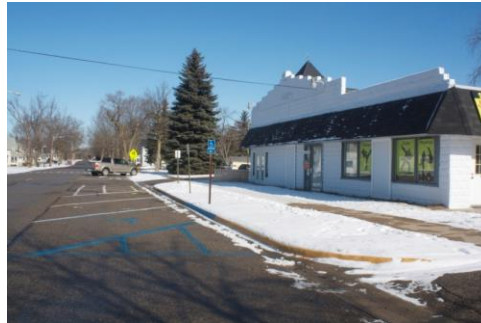
Figure 2.11. Downtown On-Street Parking
