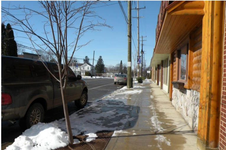
Figure 3.6. Parallel Parking Spaces on Grand River Avenue
