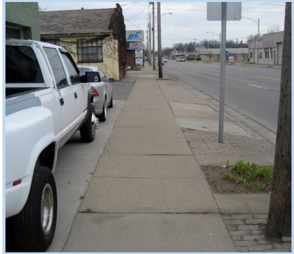
Figure 2.17- Northbound sidewalk between Paris Ave. and Denver St.
