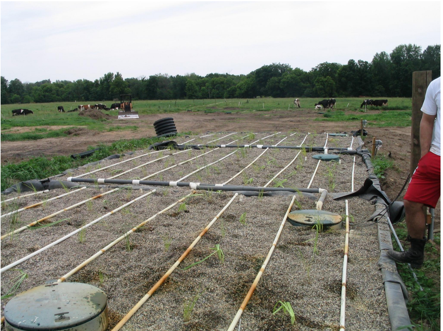
Figure 3: Surface distribution of water onto the recently vegetated VFW during warm weather season.
