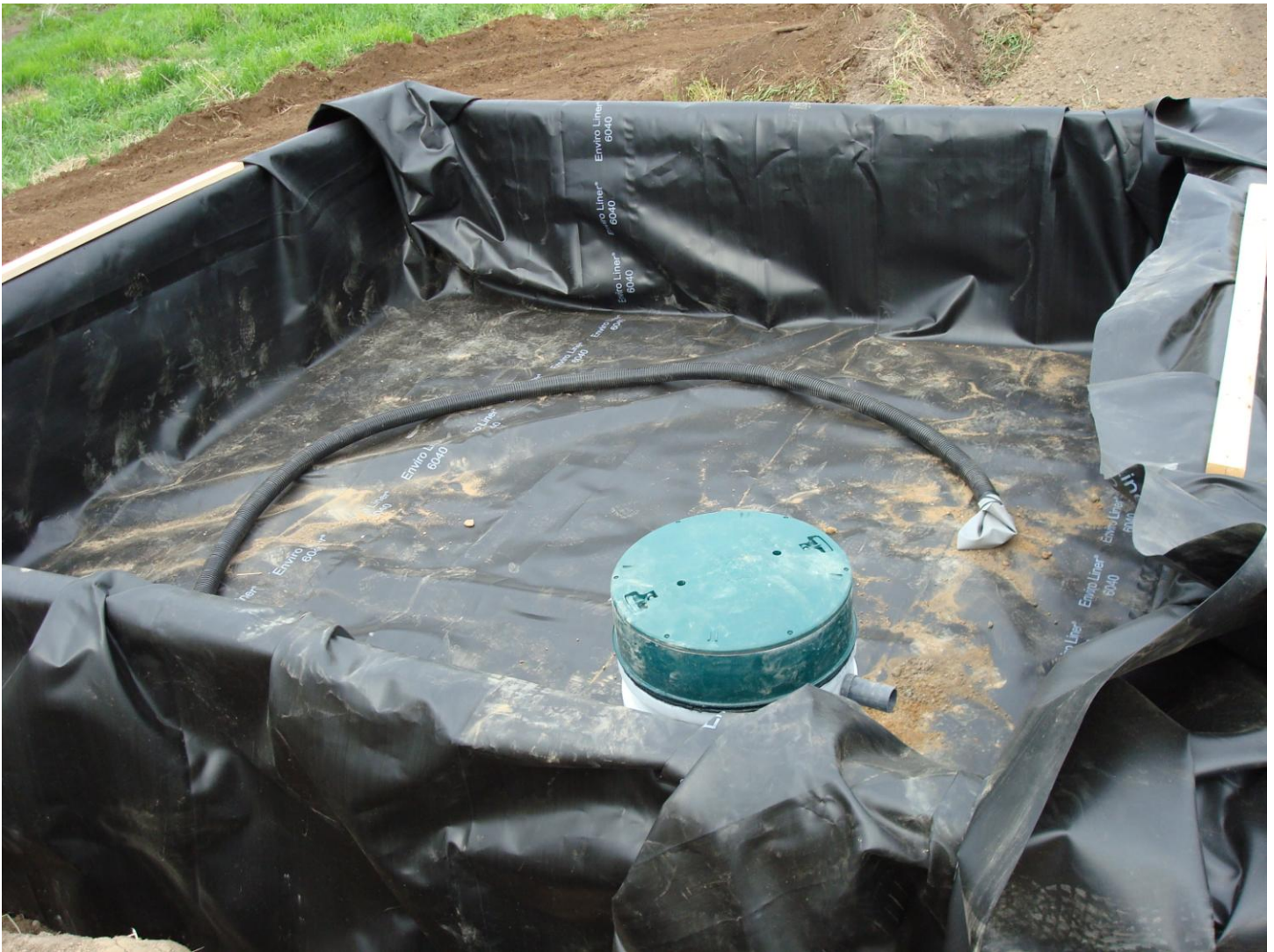
Figure 2: Empty VFW cell lined with drainage tile to collect percolated water.
