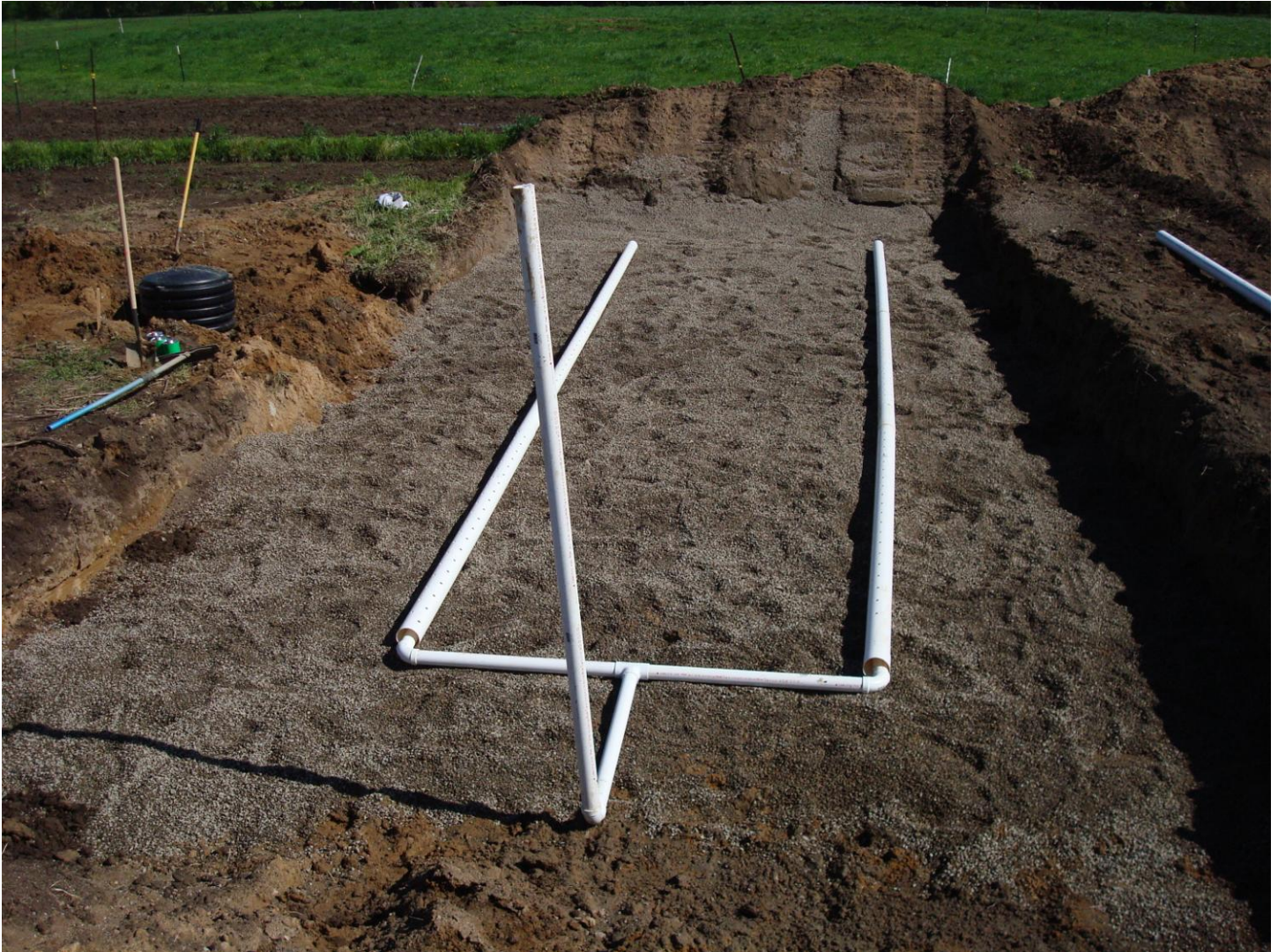
Figure 4: Drain field under construction.
