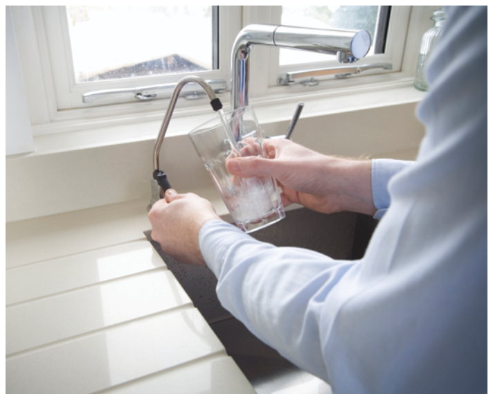
Example of a system that has separate filtered and unfiltered water options.
