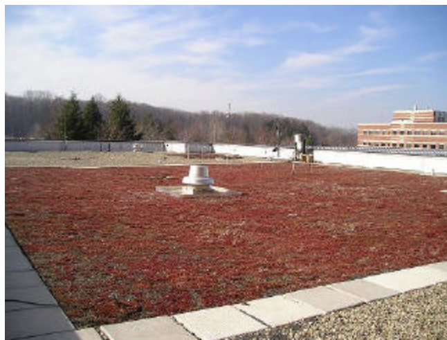
Figure 2. An extensive green roof during dormancy in East Lansing, Mich.
