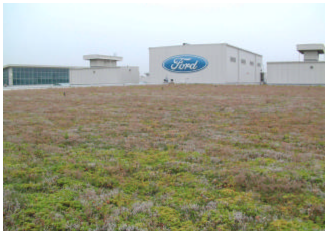
Figure 1. A 10.4-acre extensive green roof in Dearborn, Mich. at the Ford Motor Co. River Rouge assembly plant.
