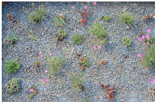
Figure 4. Green roof established with plugs.
