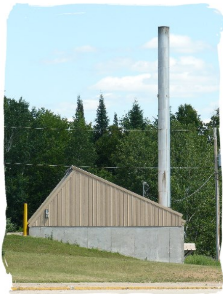
Boiler and chip storage for a school wood thermal energy system.
